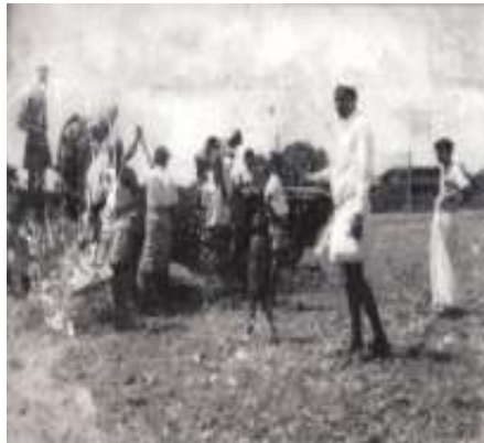
Playground in the making
